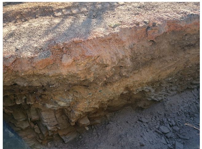
Photo 6: Trench side, rock materials.
