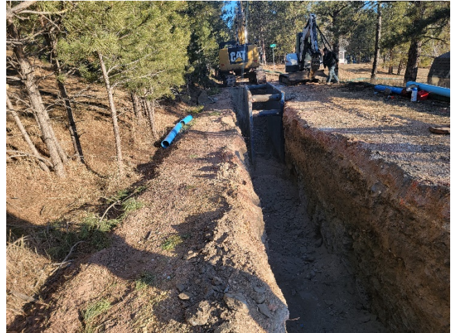
Photo 4: Open trench with trench box.
