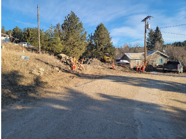
Photo 1: N 7 th St. connection point, backfilled.
