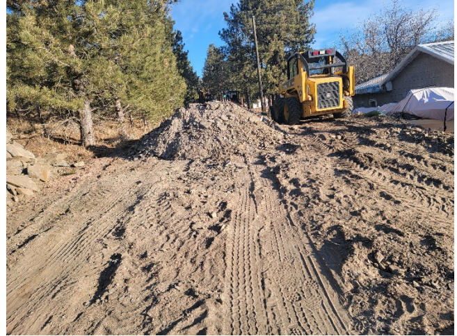
Photo 2: Some backfill material onsite from trench
