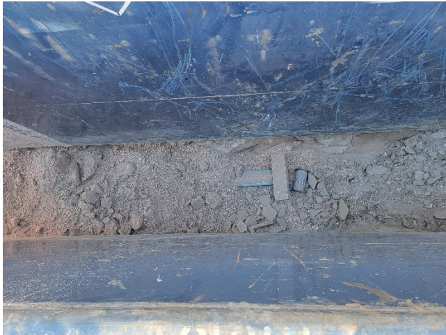
Photo 9: Water main end in trench box with bedding
