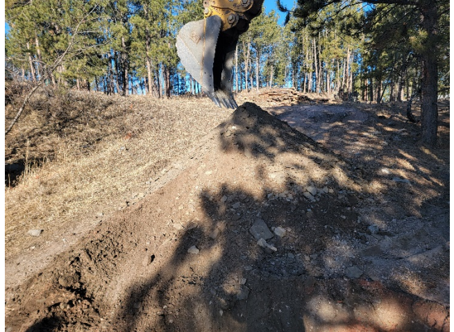
Photo 8: Trench excavation material at test hole.
