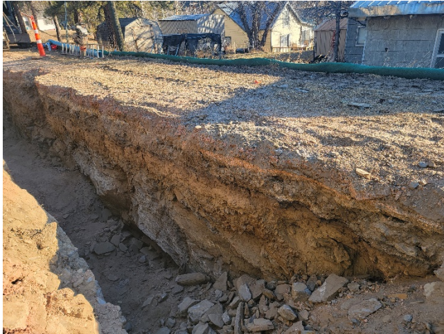
Photo 3: Excavated open trench.
